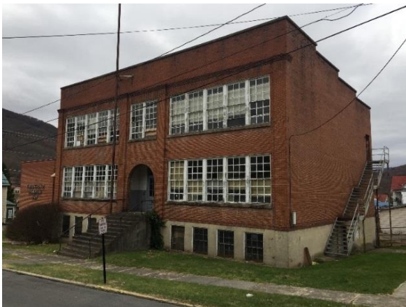
Clifton Forge East Elementary School
